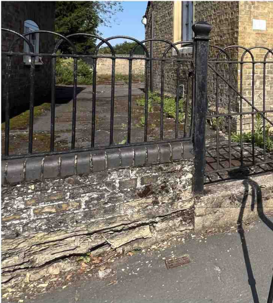
Dwarf Wall and Railings
