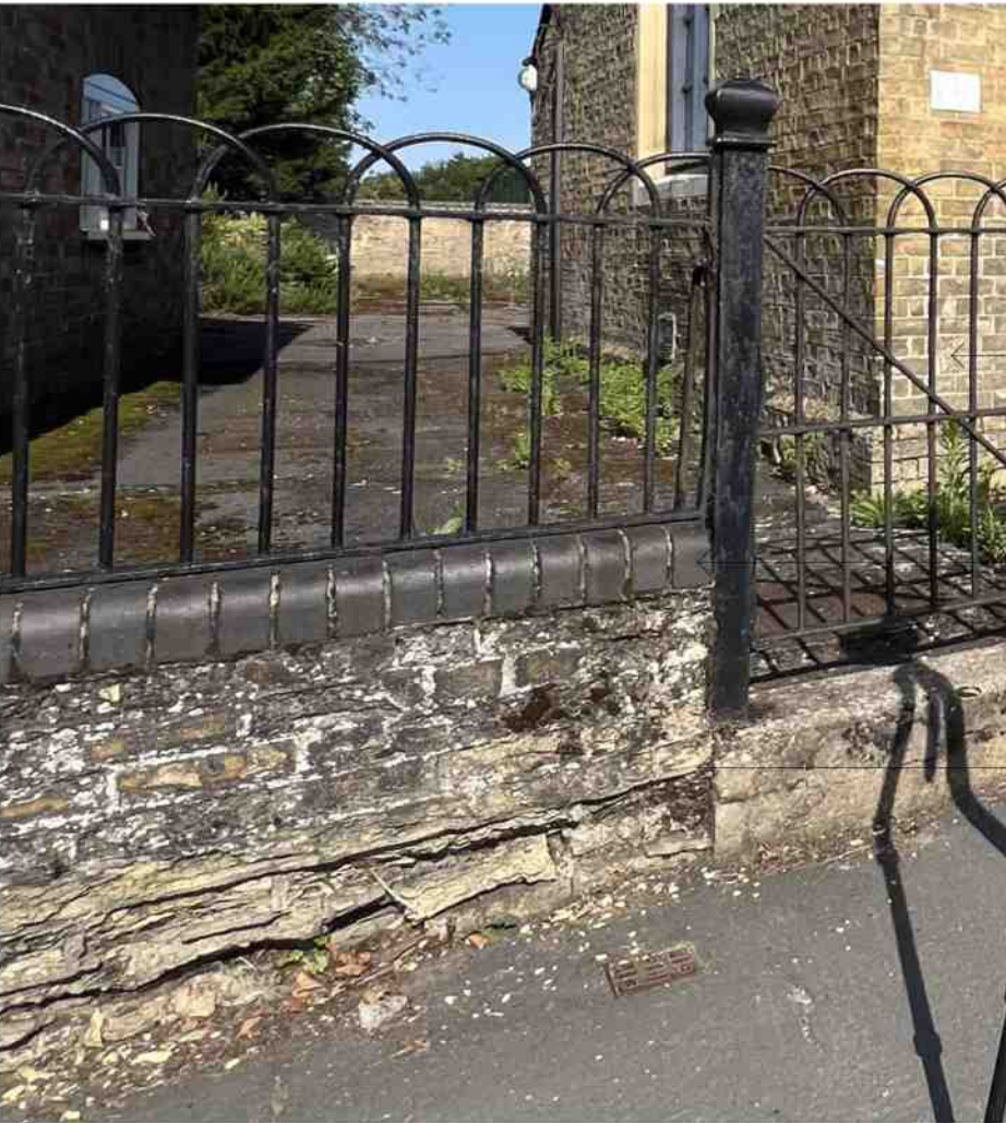
Dwarf Wall and Railings
